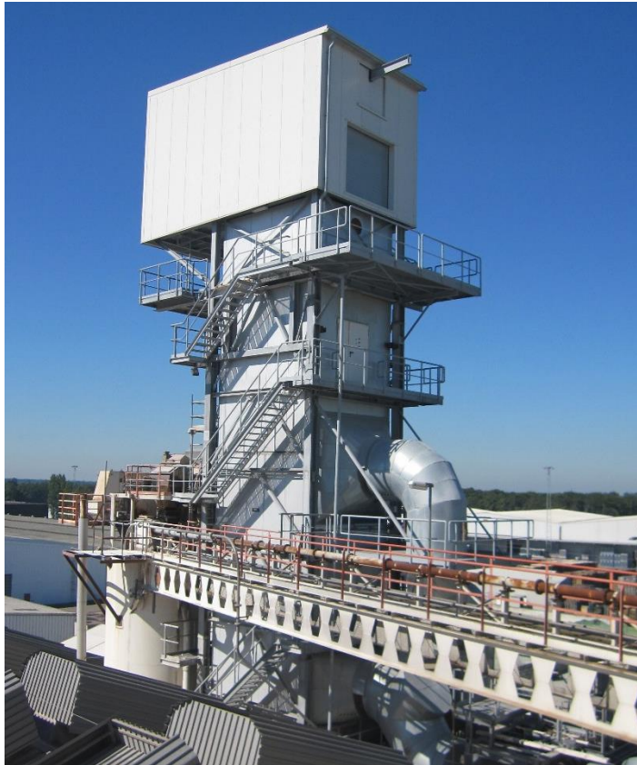
Preheating system installed in 2011
