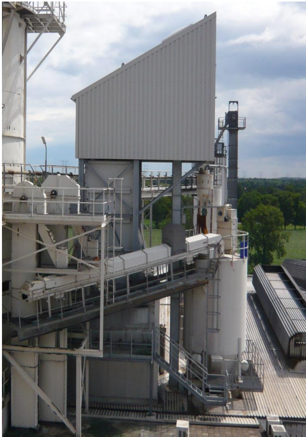
Preheating system installed in 2010
